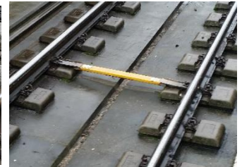
Tracklink® III Beacon Vossloh Fixing HSD2300/092 PADS 086/011796
