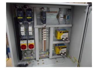
The system I/O is configured as Duplex (two channels). That is, two I/O channels are assigned to each input and output.
